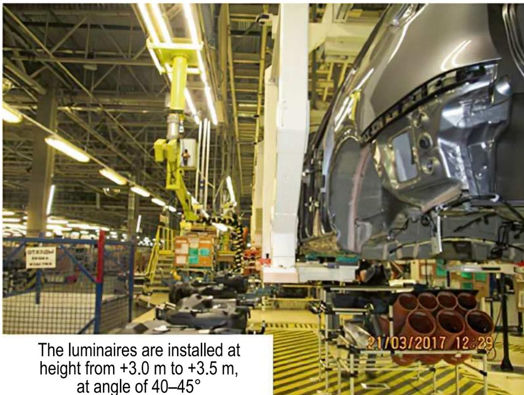
The luminaires are installed at height from +3.0 m to +3.5 m, at angle of 40–45°
