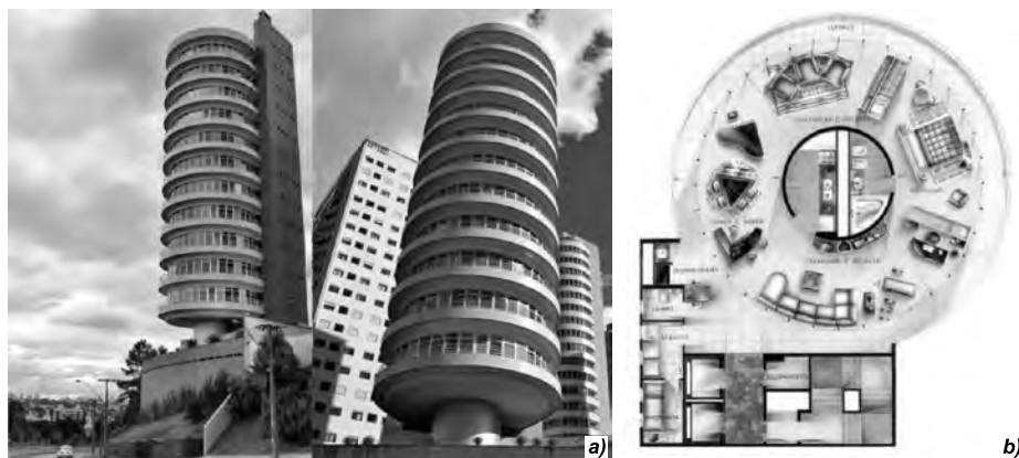
Fig. 3. The Suite Vollard turning house: a) general views; b) layout of a floor URL: http://geographyofrussia.com/krutyashhiesya-kvartiry-v-bashne-suite-vollard/
