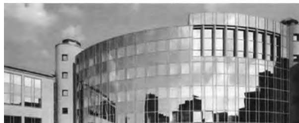
Fig. 1. Structural glazing forms an ideal specular surface of a building facade
