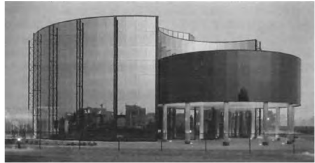
Fig. 2. Reflection of opposed buildings in a standard specular facade with transoms
