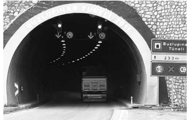
Fig. 4. Illumination of the Buzlupınar tunnel using HPS luminaires
