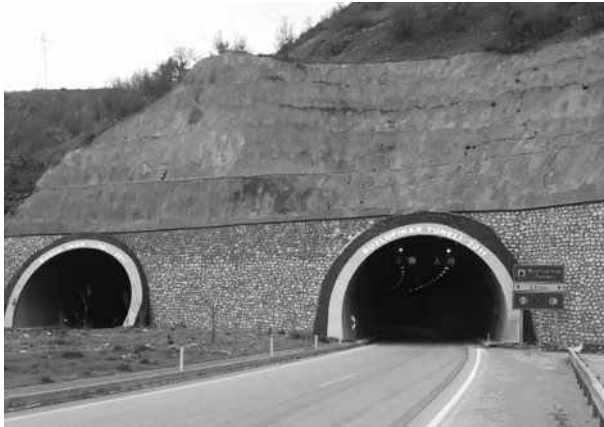
Fig. 3. Two tube views of the Buzlupınar tunnel
