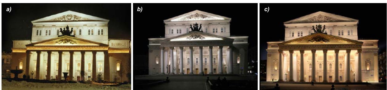
Fig. 4. Different versions of the architectural illumination of the main facade of the Bolshoi Theatre in Moscow: a – previous, b – existing, c – computer generated (A.G. Batova)
