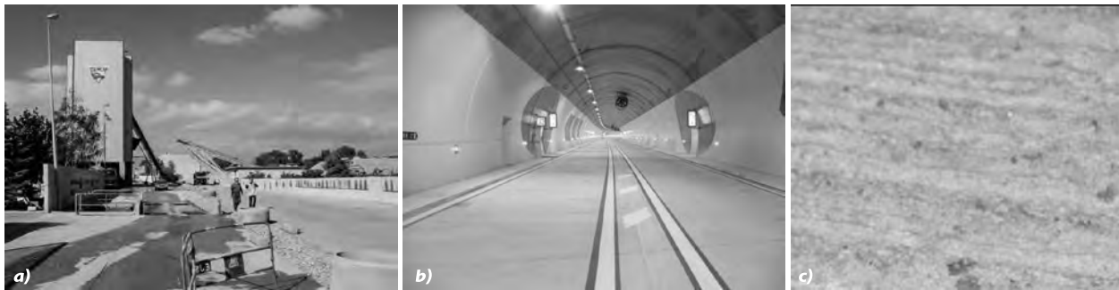
Fig.3. a) Localisation of the pilot study; b) View of the Sinarud Tunnel; c) Picture of the broomed concrete (initial state)
