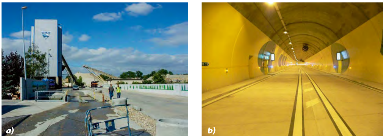
Fig.3. a) Localisation of the pilot study; b) View of the Sinard Tunnel; c) Picture of the broomed concrete (initial state)
