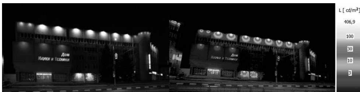
Fig.9. Evening photograph and luminance distribution over the facade, Mendeleevskaya st.1
