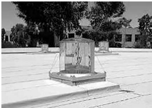
Fig. 4. *Solatube*<sup>®</sup> M74 collector of SkyVault series (740 mm) on a roof of a building. A combination of the collector and Fresnel lenses on the dome (Raybender<sup>®</sup> technology) provides constancy of luminous flux within all light day, including morning and evening periods due to catching light rays at low angles of the sun above the horizon
