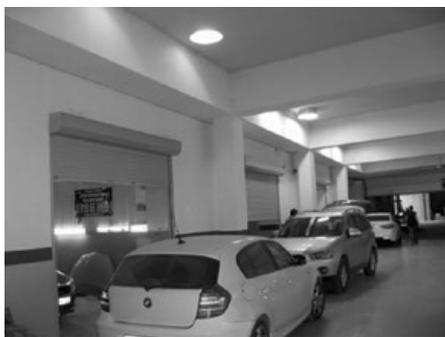
Fig. 9. *Solatube*® 330DS model illuminating underground car service centre of the KIA car dealership (Sochi)
