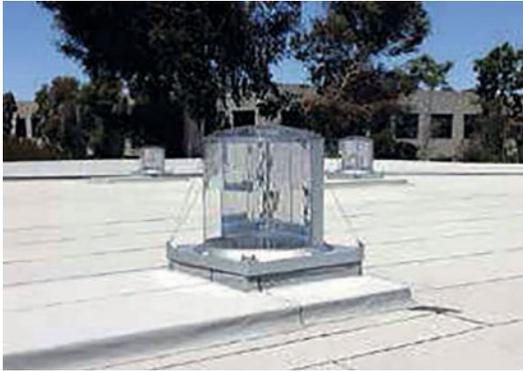
Fig. 4. *Solatube®* M74 collector of SkyVault series (740 mm) on a roof of a building. A combination of the collector and Fresnel lenses on the dome (Raybender® technology) provides constancy of luminous flux within all light day, including morning and evening periods due to catching light rays at low angles of the sun above the horizon
