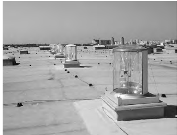
Fig. 9. General view of the FSC roof
