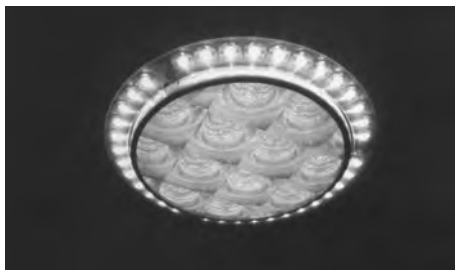
Fig. 1. LED + Solarspot hybrid illumination complex (light guide diameter is 375 mm). Installed in 2010 by Solarspot International S.r.l Company
