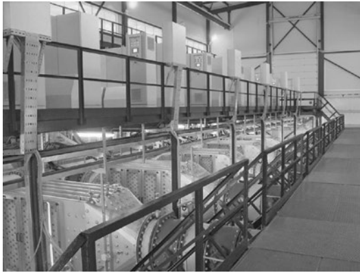
Fig. 1. UV disinfection system of the Northern waterwork (St. Petersburg) of 1,584,000 m 3 /day productivity (number of lamps type ДБ 350 is 3888 with total power consumption equal to 1.36 MW)
