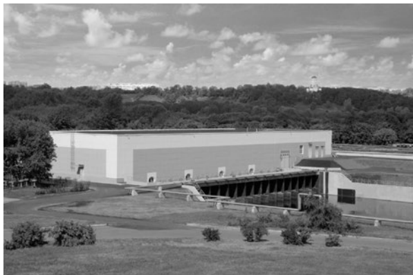
Fig. 3. UV disinfection station of the Kuryanovsky treatment facilities (Moscow); number of lamps type ДБ 600 is 6120, total power consumption is 3.7 MW
