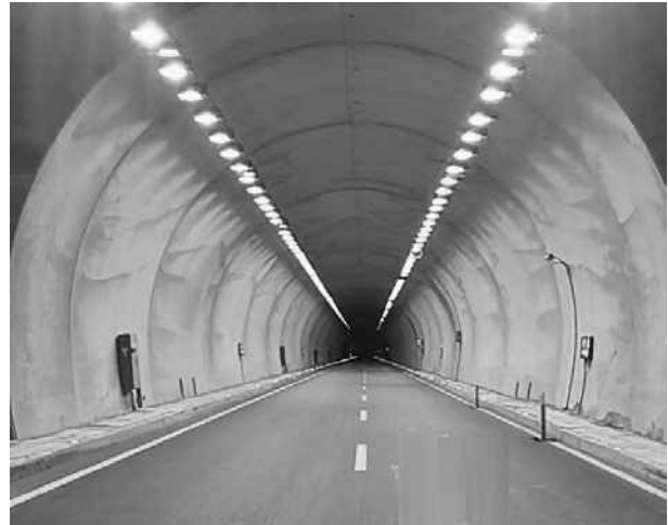
Fig. 1. Tunnel lighting with double suspensions
