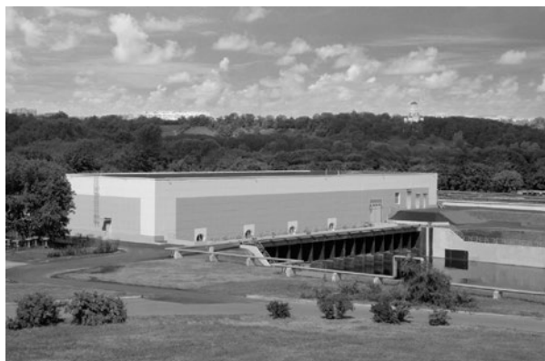
Fig. 3. UV disinfection station of the Kuryanovsky treatment facilities (Moscow); number of lamps type ДБ 600 is 6120, total power consumption is 3.7 MW
