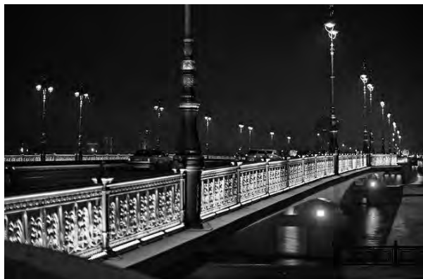
Fig. 6. Evening illumination of the Saryarka bridge. Photo of the Forbes.kz. official site http://forbes.kz/process/
