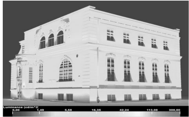
Fig. 6. Luminance distribution of the concept of floodlighting of the Rector's Palace of WUT
