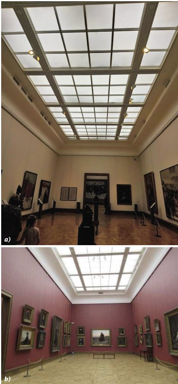
Fig. 5. General and accent lighting of the 2nd floor hall, light background (a); general and accent lighting of the 2nd floor hall, dark background (b)
