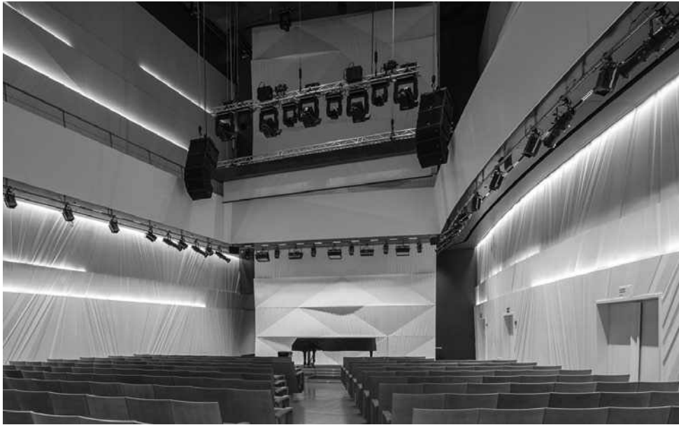
Fig. 7. Cornice lighting of acoustic panels in the small hall (photo: A. Naroditsky)
