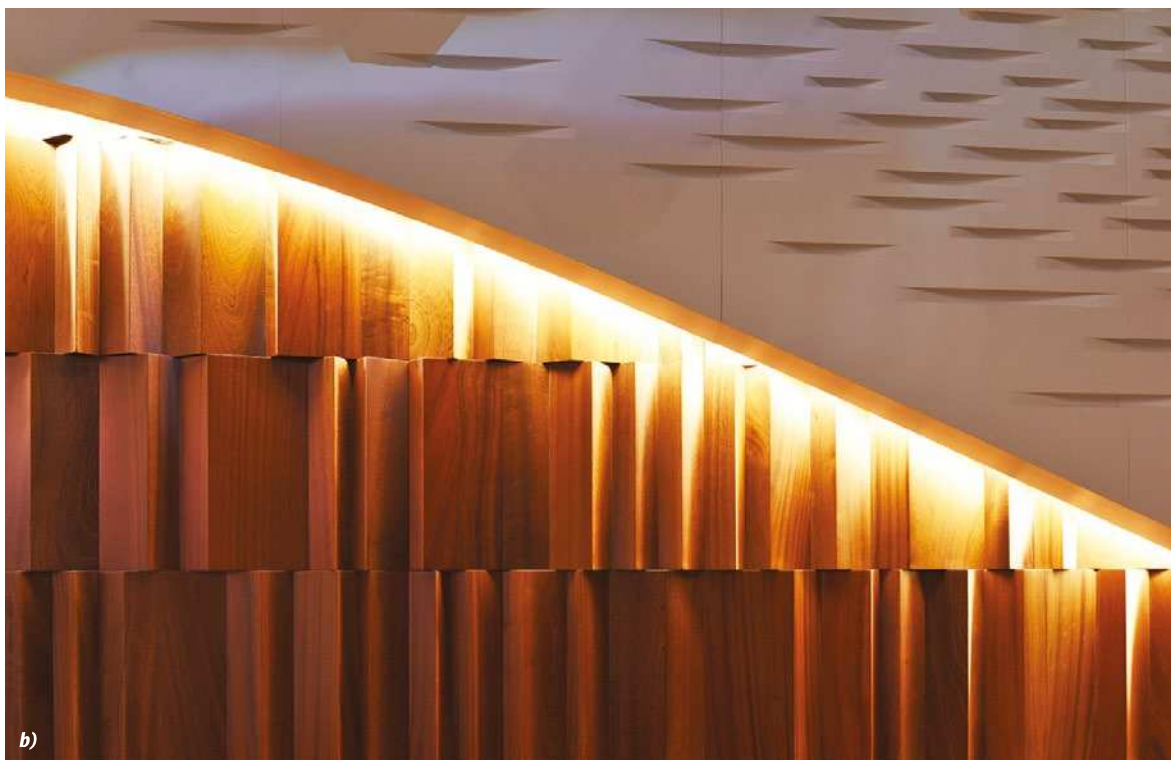
Fig. 6. Exposition of the concept idea of a layered structure in the main hall by virtue of cornice lighting: a – general view (photo: A. Naroditsky); b – “rhythmic rows” of the acoustic panel (photo: I. Ivanov)
