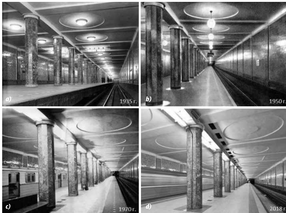
Fig. 2. Appearance of the platform at Krasnoselskaya station: (a) 1935, (b) 1950, (c) 1970, (d) 2018
