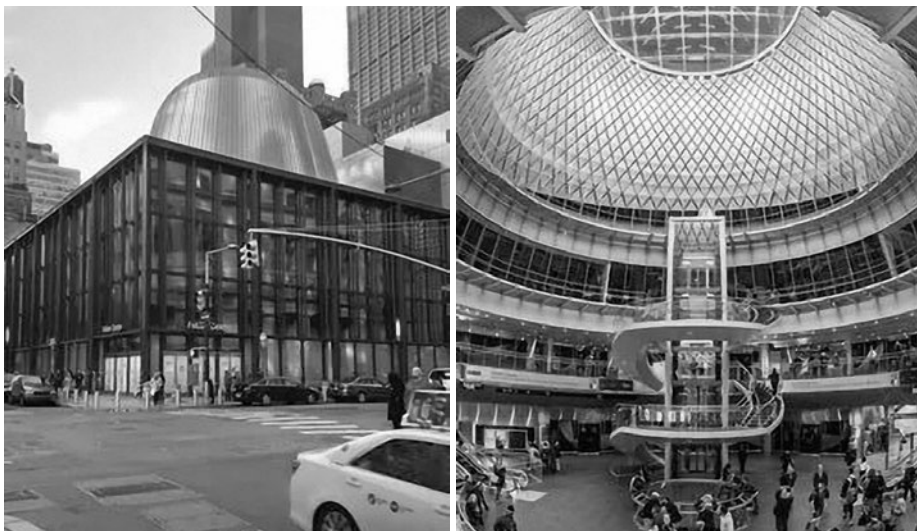
Fig.2. Trap of light in the transport interchange hub “Fulton Center”(New York): a – general view of the building node; b – internal space with a mesh structure of the dome
