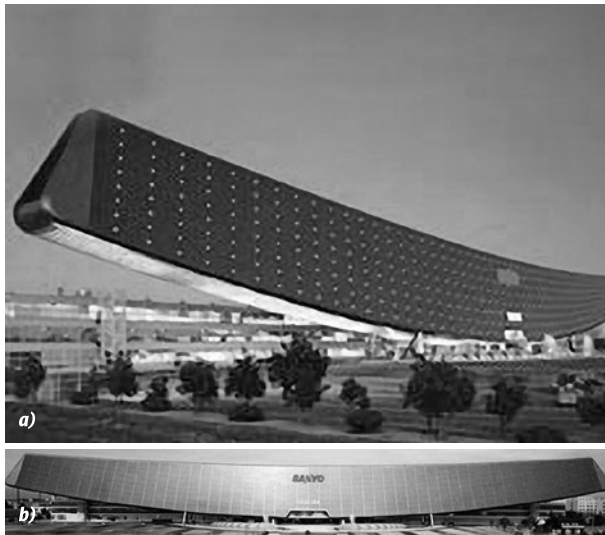
Fig. 13. Solar energy monument “Solar Ark” (Japan): a – facade; b – general view
