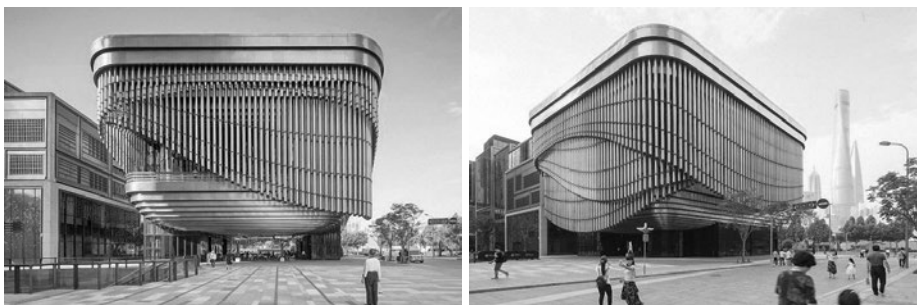
Fig. 7. Dynamic facade of the art centre in Shanghai (China): general view (transformation options)
