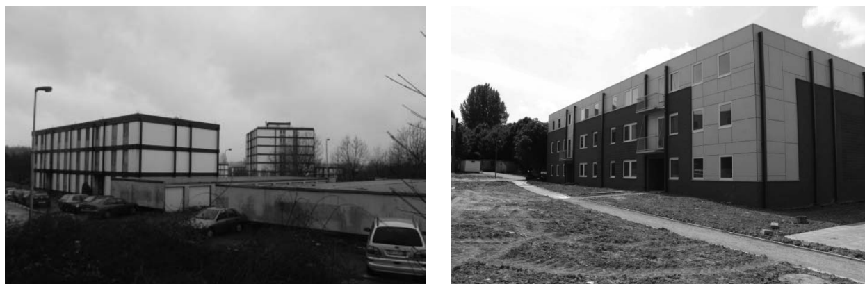
Fig. 1. View of the apartment buildings before (left) and after (right) renovation
