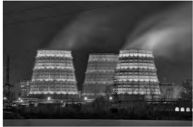
Fig. 15. Colour lighting of cooling towers CHP in Yekaterinburg
