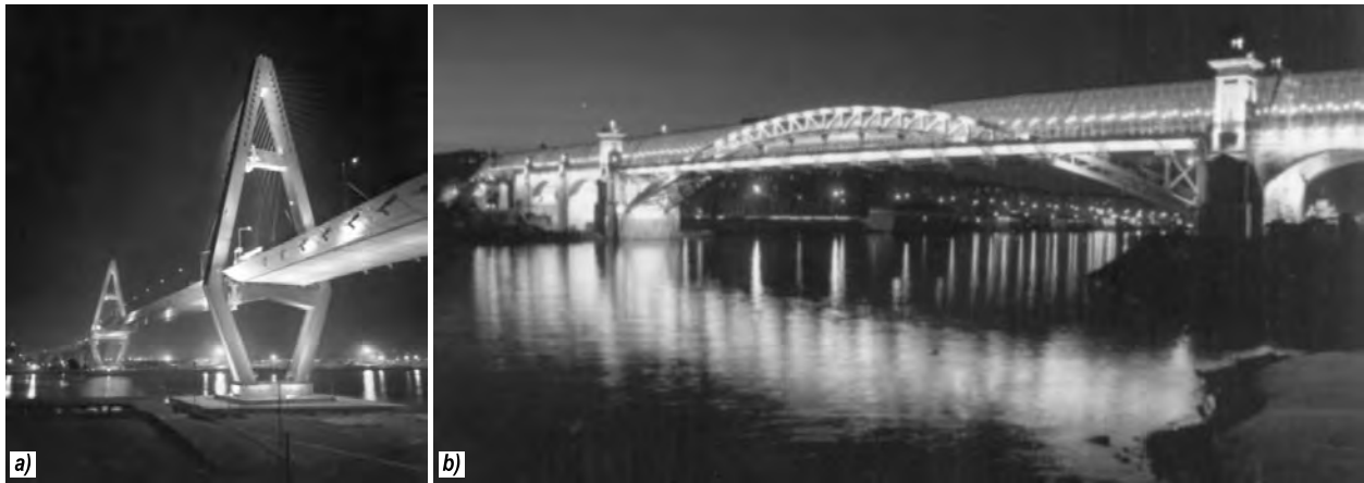
Fig. 4. Colour dynamic lighting of bridges: a – Meiko East Bridge in Nagoya; b – St. Andrew walking in Moscow (photo N. And. Shepetkov)
