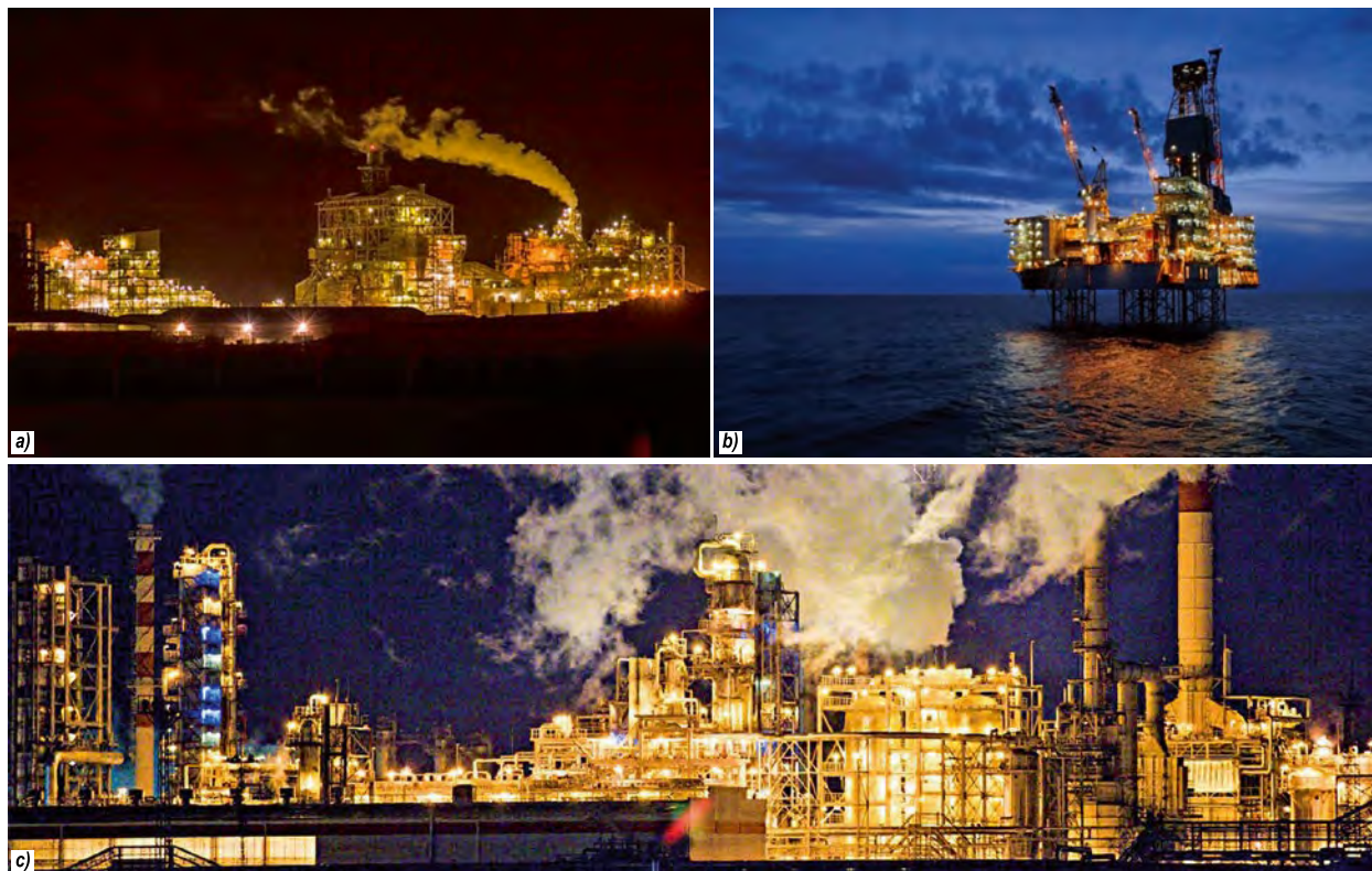
Fig. 7. Element of technical technological and signal lights in the night panoramic views of oil and gas, chemical and processing facilities:
