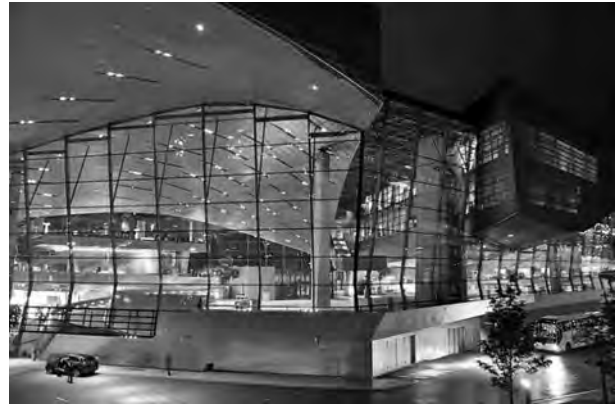
Fig.2 The glazed façade of the shop in Munich, BMW with a colour exteriorouter and interiorinner dynamic lighting in Munich
