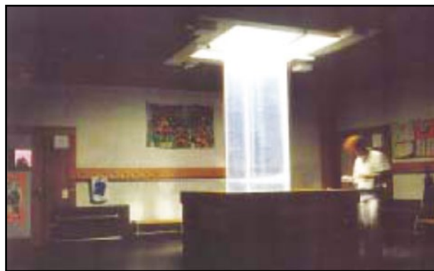
Fig. 6. View of the illuminating part of Heliobus indoors
