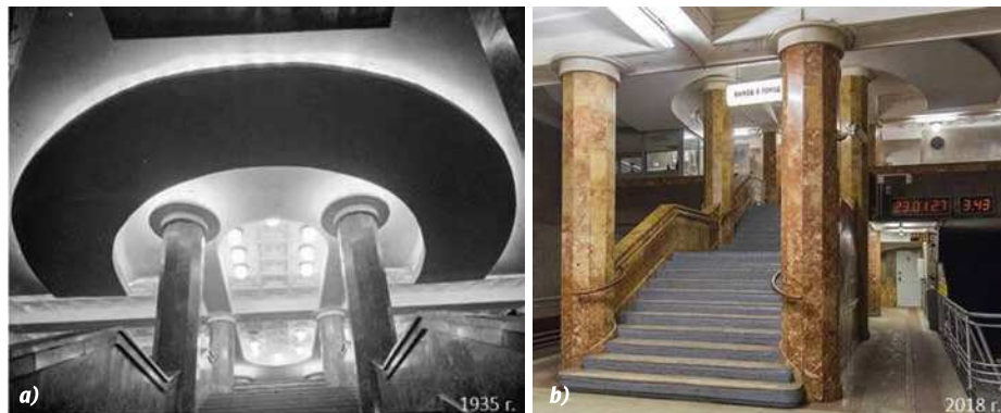
Fig. 3. Appearance of the connecting passage stairway at Krasnoselskaya station: (a) 1935, (b) 2018
