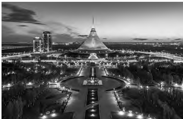
Fig. 5. An evening view of the Khan-shatyr shopping and entertaining centre. Photo of D. Chistoprudov, http://www.titus.kz/
