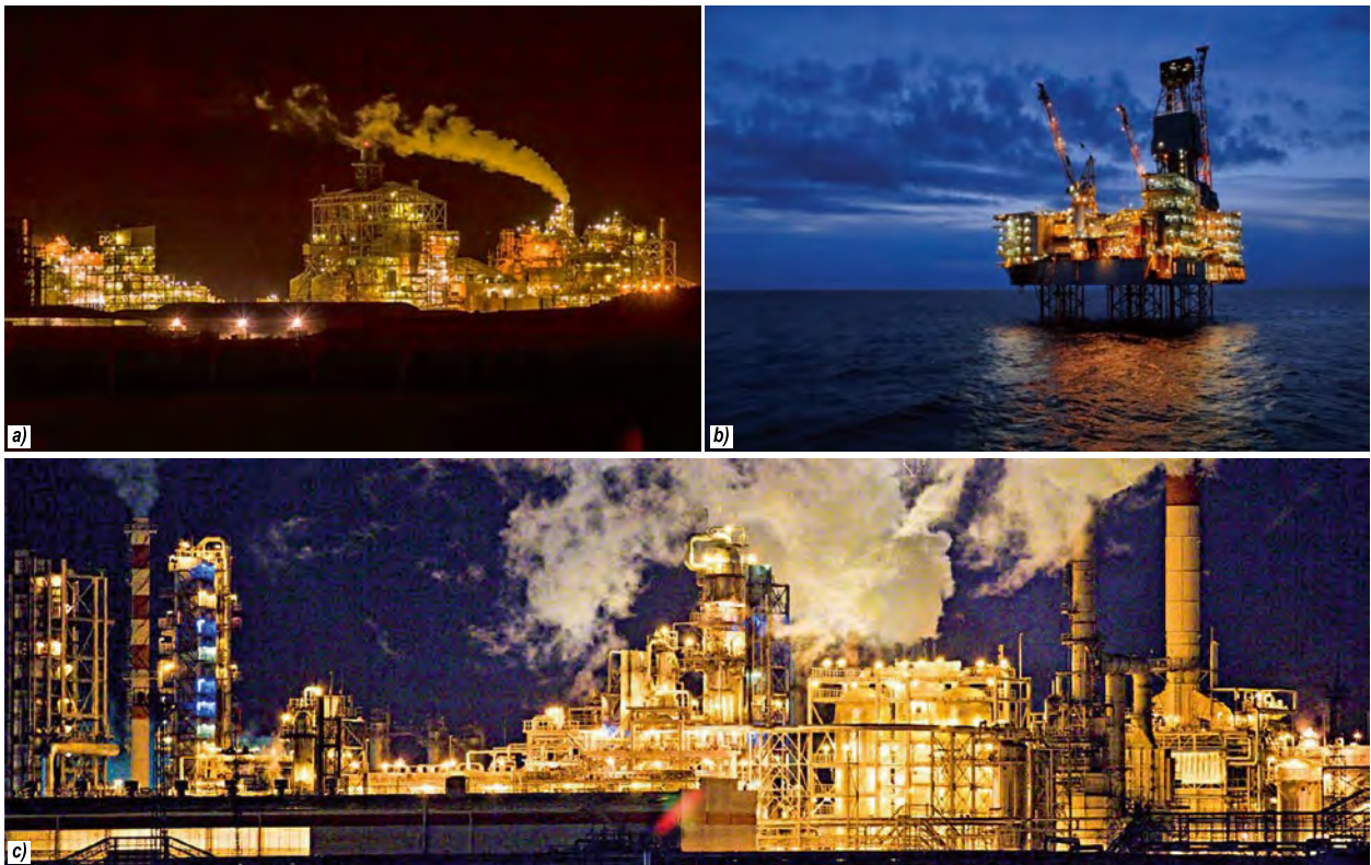
Fig. 7. Element of technical technological and signal lights in the night panoramic views of oil and gas, chemical and processing facilities:
