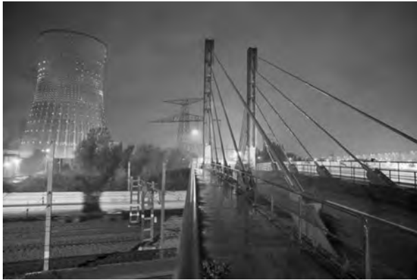
Fig.14. Lighting of the thermal power plant cooling tower in Brussels – one of the first media installation at the industrial facility
