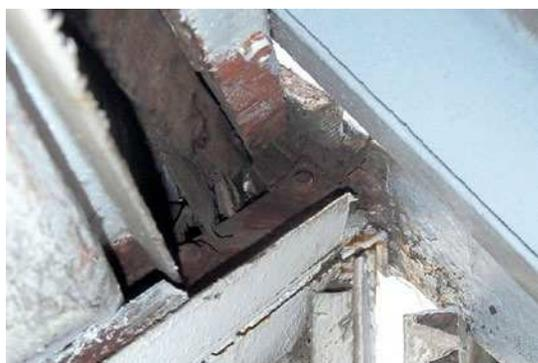
Fig. 4. Roof beam joint with traces of corrosion
