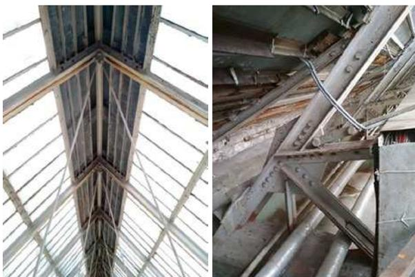
Fig. 8. Ridge of the lantern light transparent structure and traces of repairs
