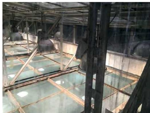
Fig. 11. Exterior of the diffusing ceiling with the lighting devices
