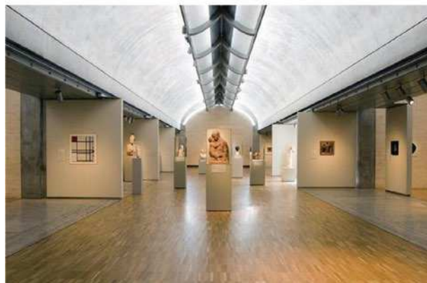
Fig. 11. Kimbell Museum in Fort Worth, Texas (L. Kahn, 1966–1972). Vaulted reflective roof and linear suspended light scattering device turn bright sunlight into a soft diffuse light in the exhibition halls. Section, day interior
