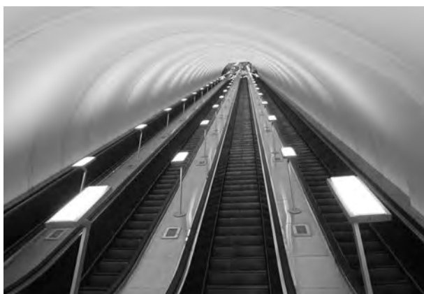
Fig. 3. Arrangement of escalator area illumination at Sretensky Boulevard station
