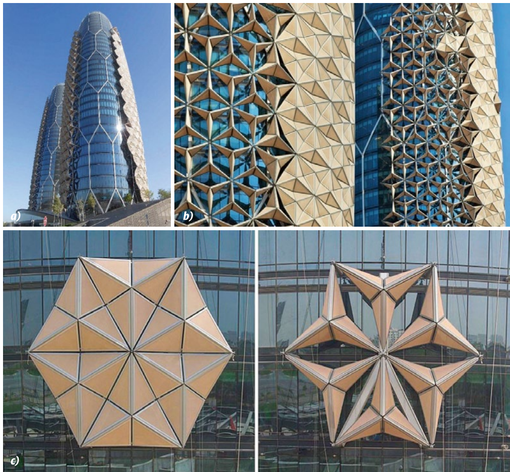
Fig. 6. The system of sun protection in the office towers “Al Bahr” in Abu Dhabi: a – general view; b – modification of sun protection devices; c – transformation scheme panels
