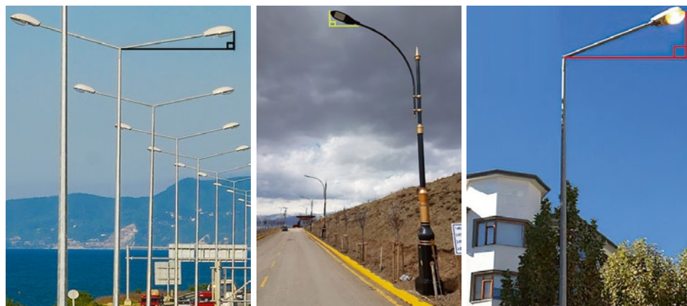
Fig. 1. Examples of road lighting console angles
