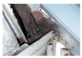
Fig. 4. Roof beam joint with traces of corrosion
